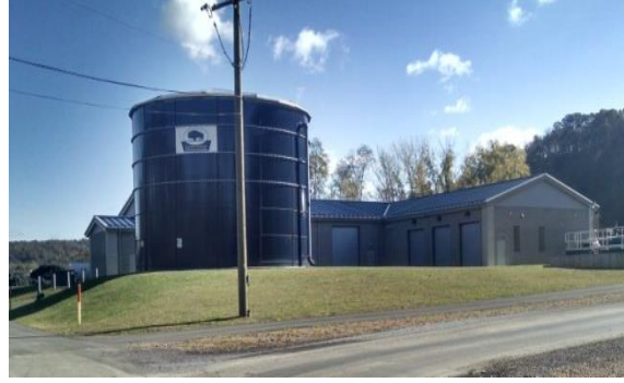
The Stanley K. Swank Freeport Filter Plant
